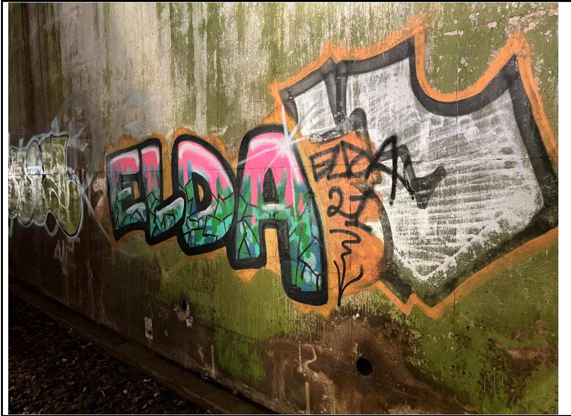
1717_P26_2024 West abutment - Drainage weepholes
