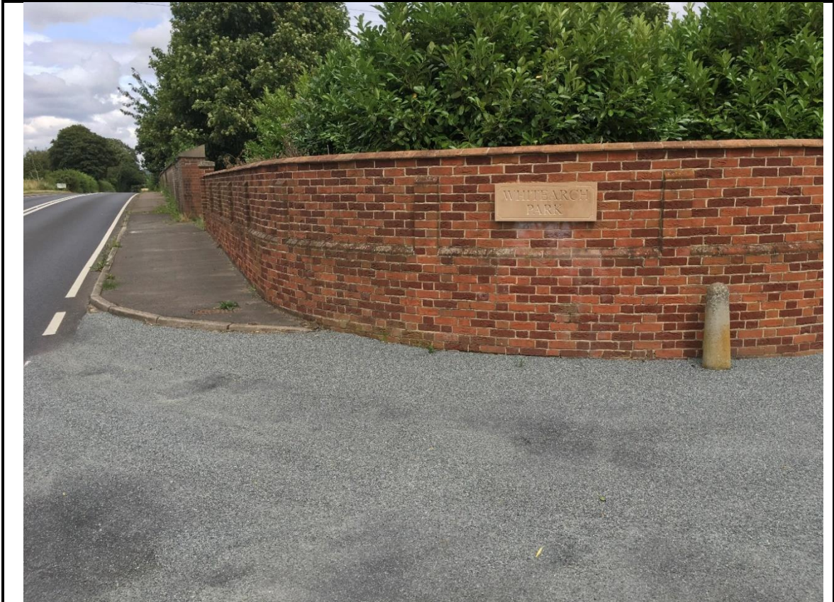
1717_P44_2024 – South footway - Footway surfacing (July 2023)
