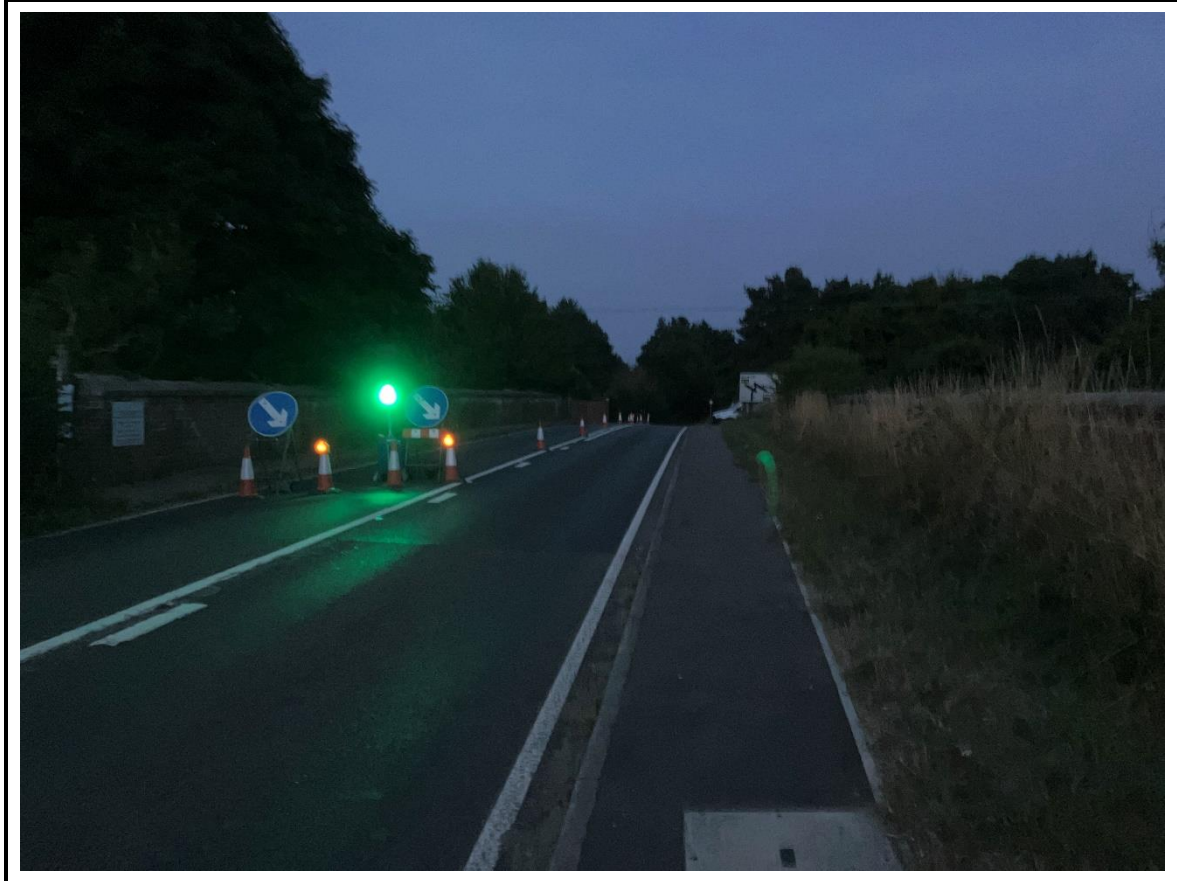
1717_P42_2024 West view - Carriageway
