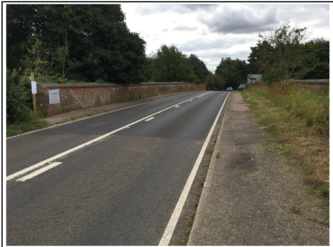
1717_P4_2024 Approach looking West (Image captured 19/07/23)
